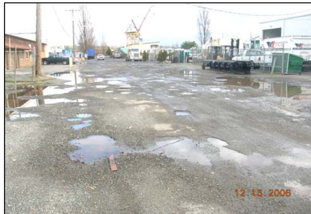
Figure 2. Typical industrial street area in the lower 7th Ave S basin
